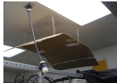
Figure 12: Homemade Airflow Shield
