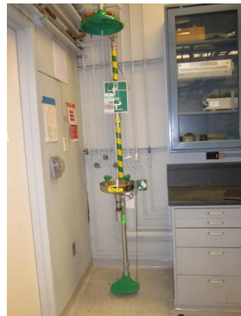
Figure 13: Eyewash Shower in Lab, Good Location
