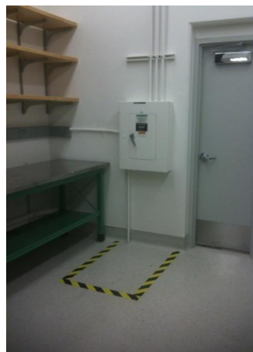
Figure 14: Clear Space Around Electrical Panel
