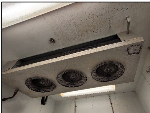
Mould growth on ceiling and fan unit in cold room
