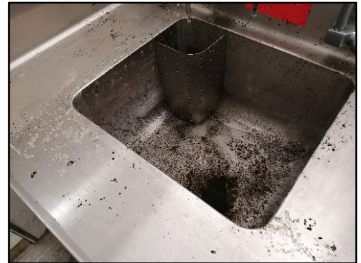
Mould growth on cold room sink and countertop
