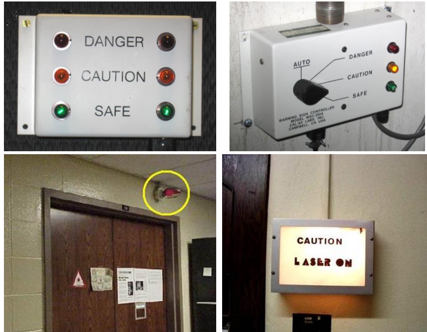
Figure 7-24: Three colours laser sign for class 4 lasers (top-left) and its control system (top-right). Other types of common laser lights (bottom row).
