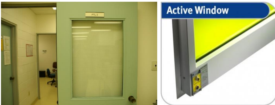
Figure 7-19: Window protection, non-transparent cover (left). Window protection with adequate OD for the laser wavelength (right).
