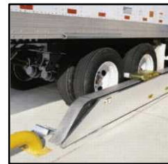
Vehicle Restraint: Automatic Wheel Type
